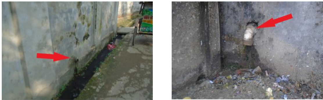
Figure 5: Containment technologies and their connections in Jamalpur. Left: Septic tank connected to nearby water body. Right: Toilet pipe connected to open drain.
