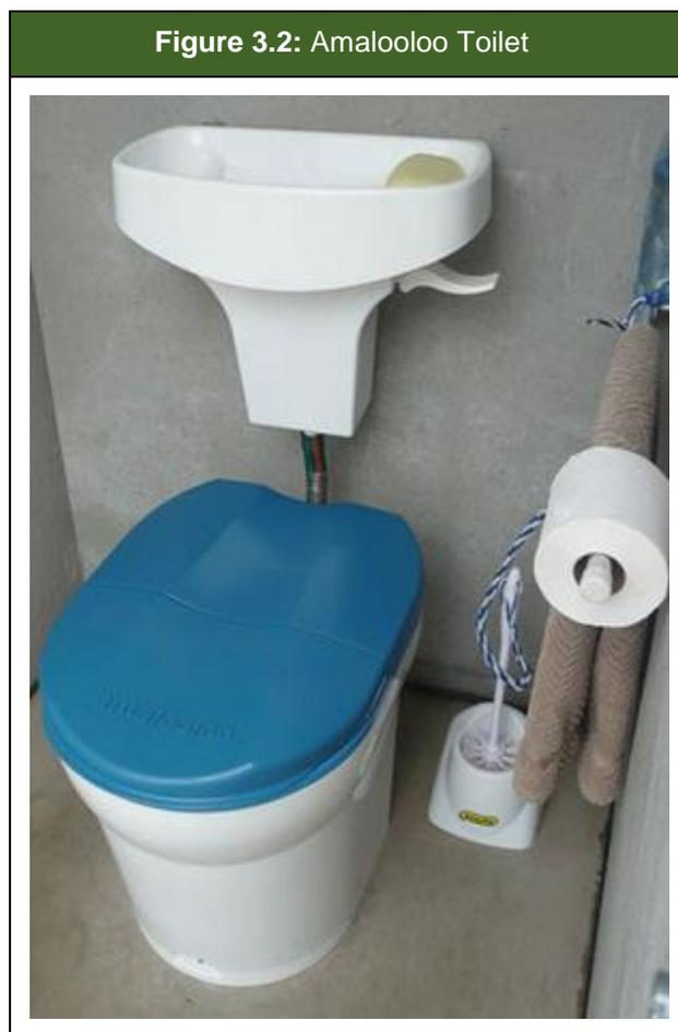
The innovatively designed Amalooloo Urine Diversion System allows for liquid separation at the bottom of the pedestal without any issues of blockage.
