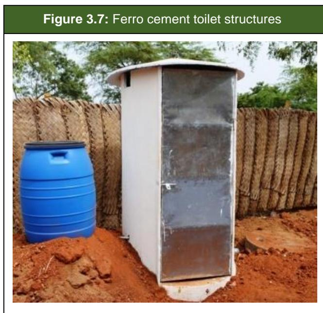
Casting at a central location takes advantage of economies of scale thereby reducing manufacturing cost. Transportation costs are also kept minimal due to the small size of modules and less weight, making these an ideal alternative for low cost toilet construction.
