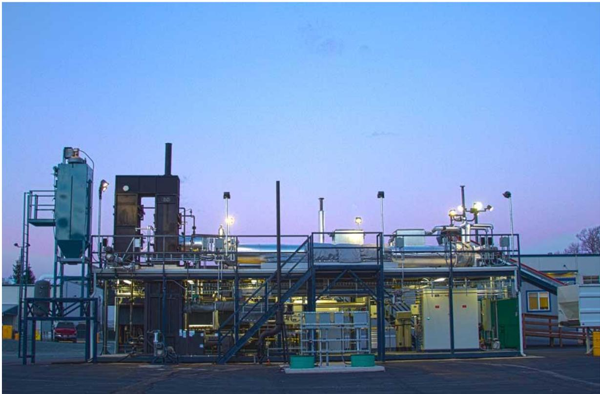
Heat generated from combustion within a fluidised sand bed is utilised to generate high pressure steam expanding in a reciprocating piston steam engine connected to a generator and producing electricity. The exhaust (process heat) from this engine is used to dry the incoming faecal sludge. Water evaporated from the
