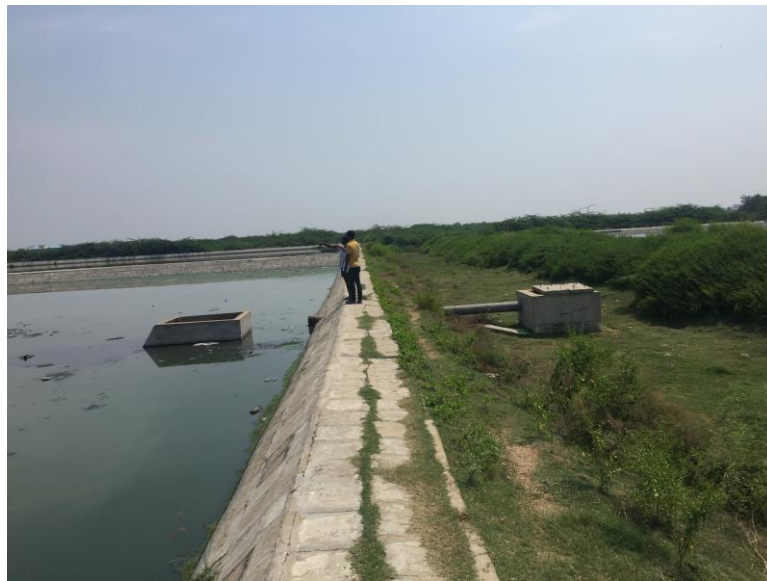
Figure 1.20: Waste Stabilisation Pond at Kancheepuram
