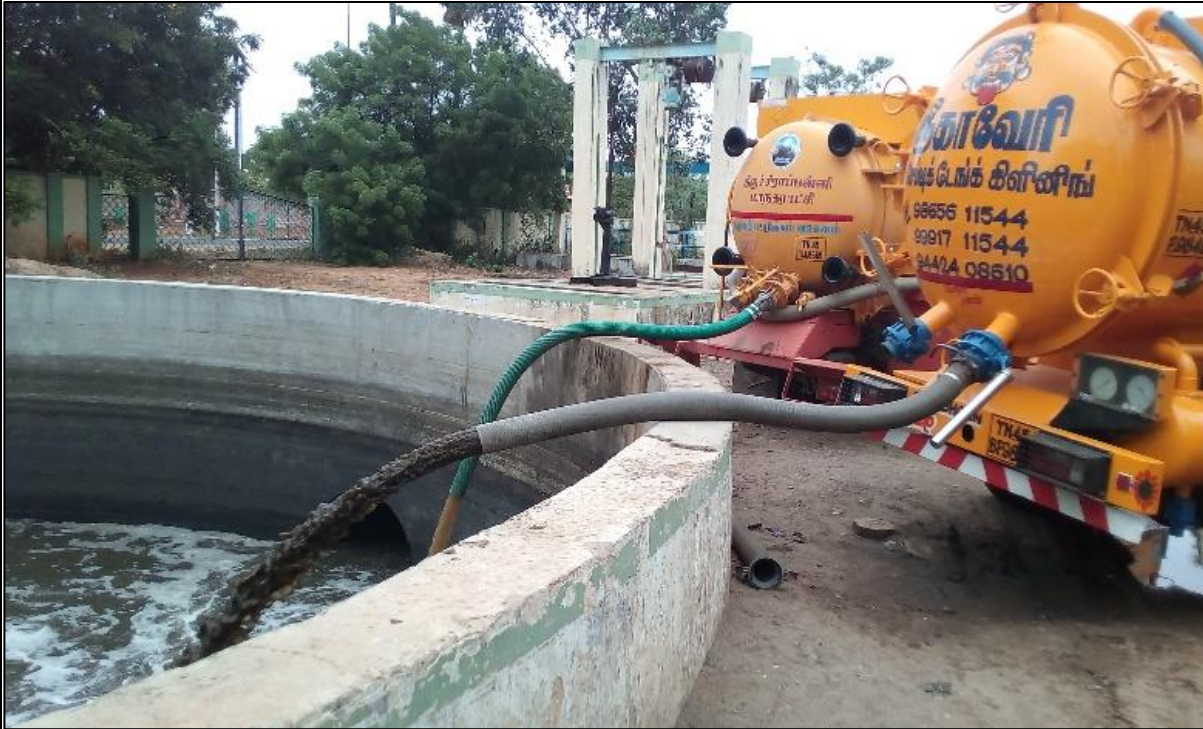
Figure A2.1: Photos of emptying FS/septage into collection well
