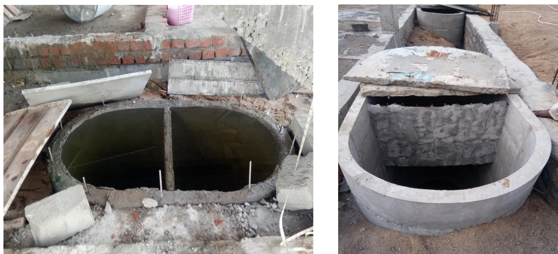
Figure 4: Elliptical septic tanks with partition wall built in Sircilla.
