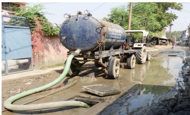
Figure 1: Vacuum tanker is used for unclogging sewers (Source: Bhavik/CSE, 2016)
