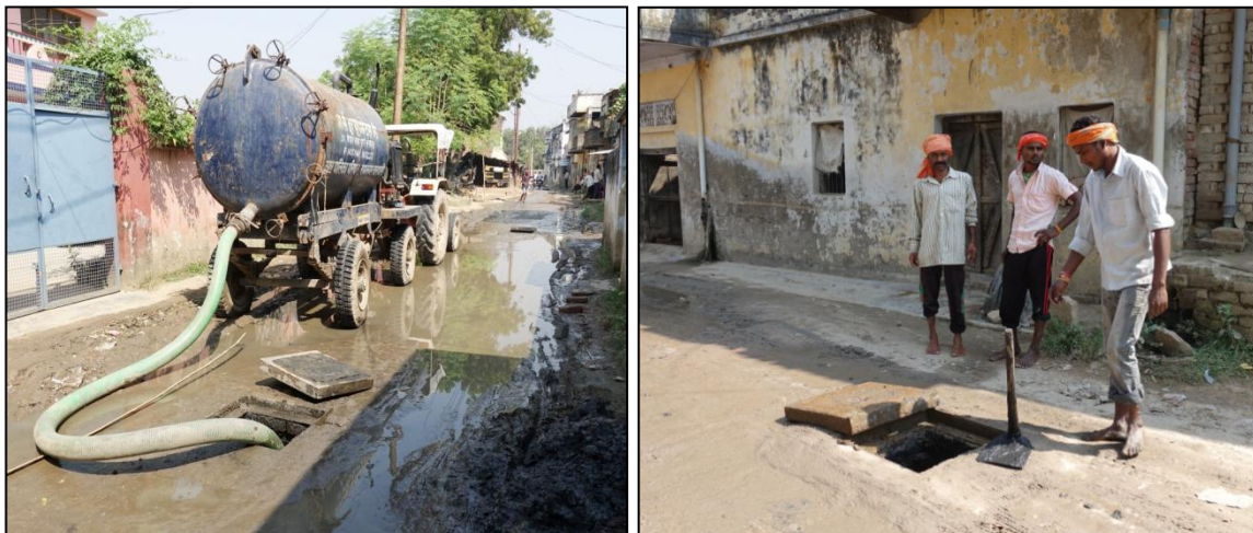
Figure 3: Vacuum tanker is used for unclogging sewer manholes (Source: Bhavik/CSE, 2016)
