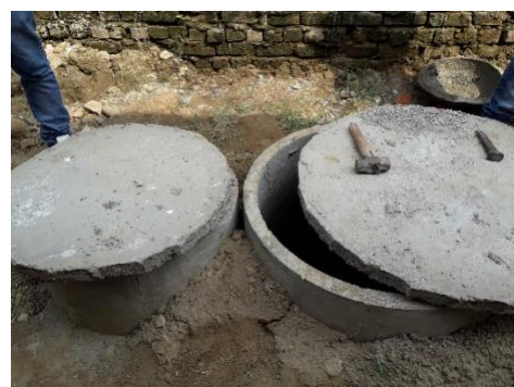
Figure 5: Septic Tank in under construction house (Rahul/GIZ, 2018)
