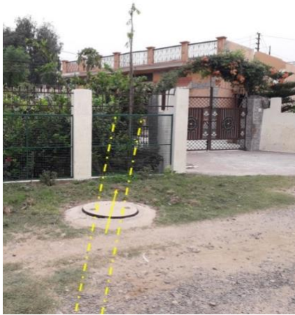
Figure 4: Settlements constructed over trunk sewer in Nirmal Block (Rahul/GIZ, 2018)
