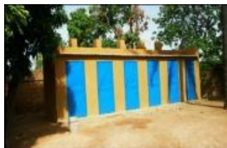
Figure 4: Public facility constructed by ONEA
