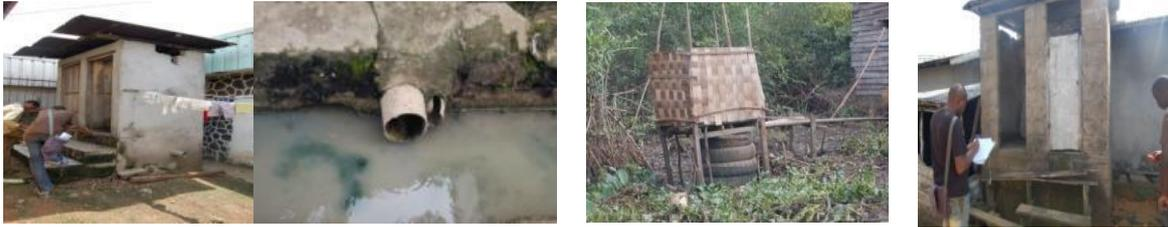
Illustration of a lined tank with hole towards water body (the content of this type is emptied to the water body)
