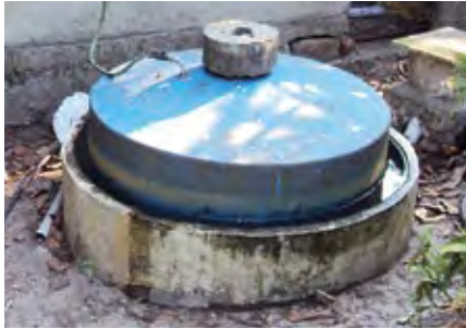
Picture 17: Steel floating-drum with water jacket and weight on top of the drum (photo: Sandec).
