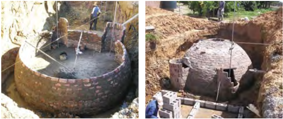
Picture 9: Fixed-dome digester under construction in Lesotho (photo: Sandec).
