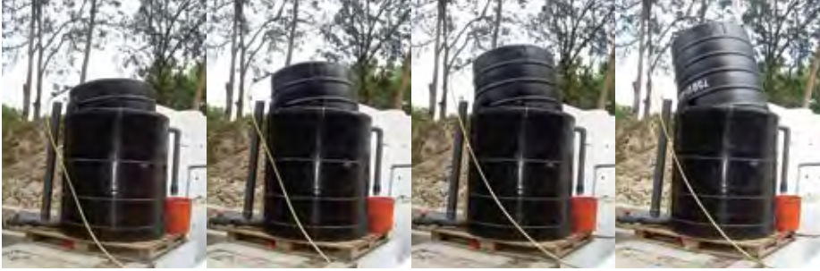
Picture 16: Rising floating-drum with increased gas production. ARTI system, Tanzania (photo: Sandec).
