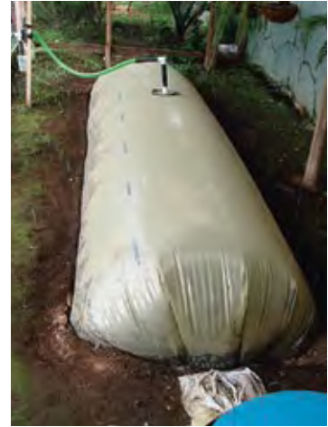
Picture 13: Tubular digester in Costa Rica (photo: Sandec).
