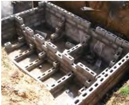
Picture 34: Anaerobic baffled reactor under construction. TED-BORDA Lesotho (photo: Sandec).
