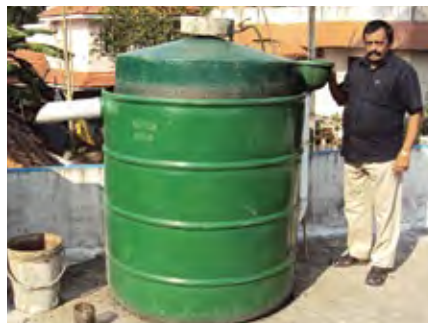
Picture B5: Newer model made completely out of Fibreglass Reinforced Plastic (FRP) (photo: Sandec).
