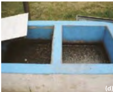
Picture H1: a) Schematic of horizontal plug-flow digester at Emilia, b) and c) Overview of AD plant, d) Outlet of anaerobic digester, e) Gas holder (photo: Eduardo S. Groppelli).
