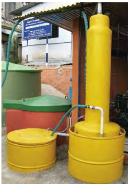
Picture 25: Biogas scrubber to remove \text{H}_2\text{S} at BIOTECH, India. The gas flows upwards through a column in which water containing iron salts is circulating in counter current. The \text{H}_2\text{S} is dissolved in the water and oxidised (photo: Sandec).
