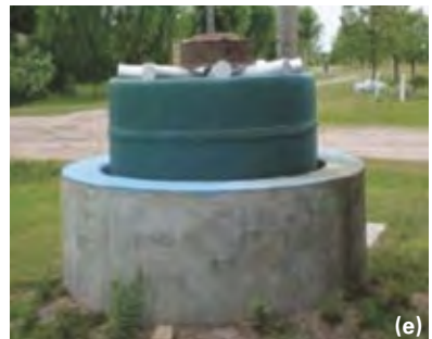
Picture H1: a) Schematic of horizontal plug-flow digester at Emilia, b) and c) Overview of AD plant, d) Outlet of anaerobic digester, e) Gas holder (photo: Eduardo S. Groppelli).
