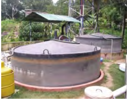
Picture 10: Floating-drum digester for market waste in India (photo: Sandec).
