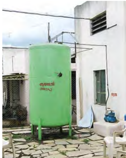
Picture 20: Gas tank in India with 10 bar pressure (photo: Sandec).
