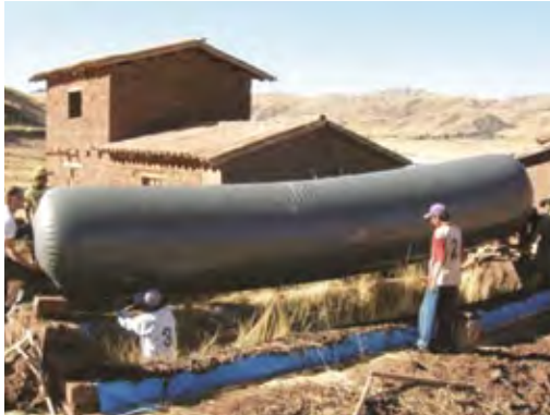
Picture 12: Tubular digester in Yanaoca, Cuzco (photo: Herrero, 2007).
