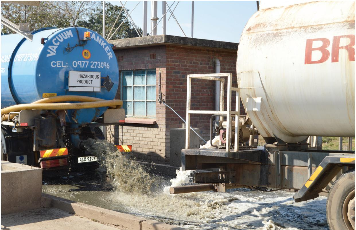
Figure 2: Tankers discharging faecal sludge
