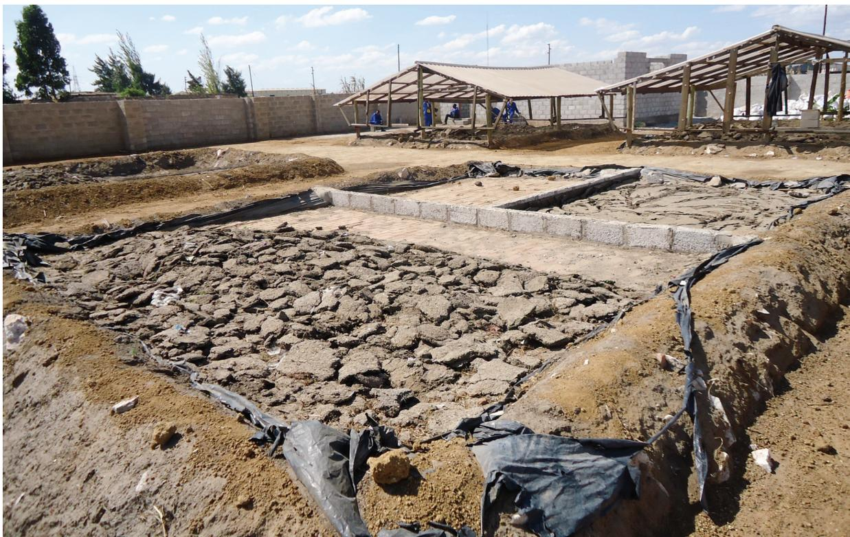
Figure 6: Sludge drying beds
