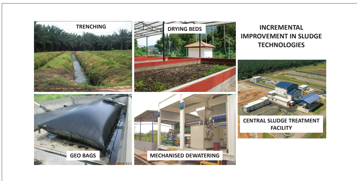
Figure 6: Incremental improvements in sludge treatment technology
