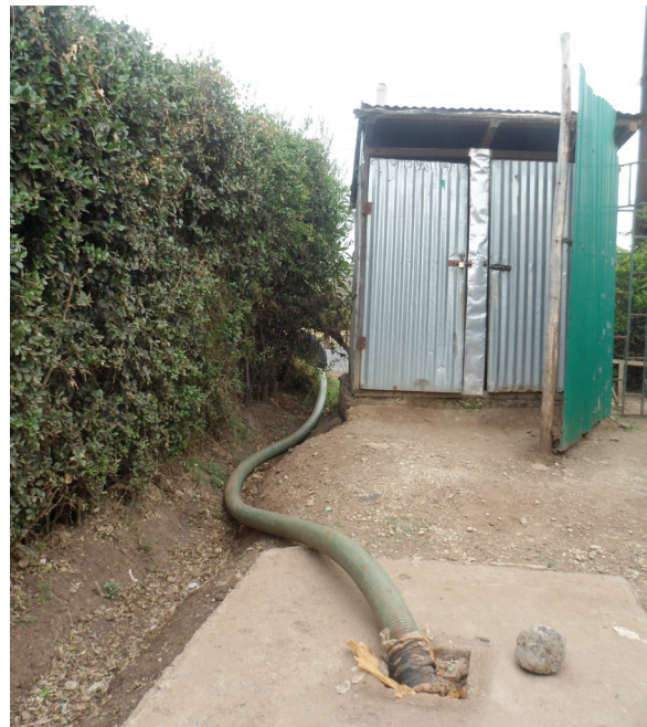
Figure 2: Septic tank being emptied by a vacuum truck ©GIZ/Doreen Mbalo
