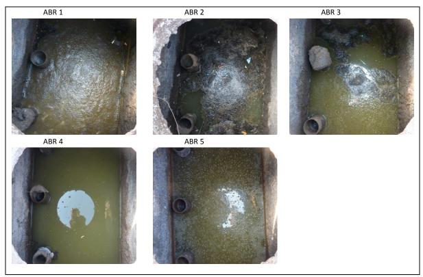
Figure 116 a, b, c, d and e: photographs taken through the ABR manholes showing chamber supernatant and down flow pipes, photographed on 26.08.2013
