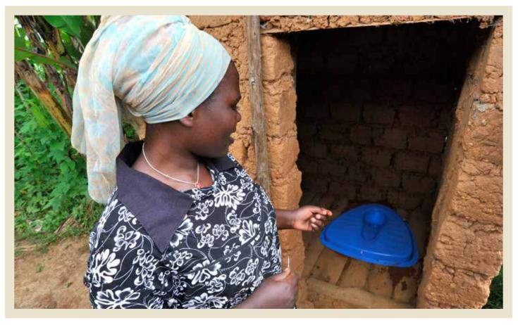
A prototype of the new American Standard plastic slab with SaTo pan fitted in an existing latrine in Rwanda.
