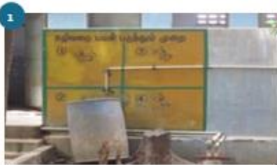
Construction of indiv/shared / community toilets financed by MFI
