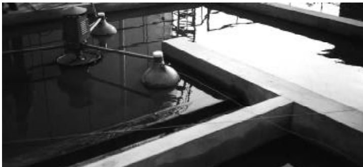
Fig. 1. One of too many non-aerating aerators [photo: Sasse]
