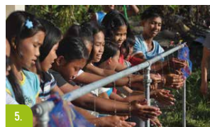
5. Punched water pipes with 1.5 mm holes reduce costs, water consumption and are more durable compared to faucets.
