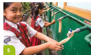
8. Make sure that children can comfortably reach the flowing water. Check the height and width of the basin.
