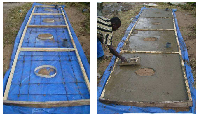
Fig. 5: Fossa alterna slabs during construction (source: ROSA Project, Arba Minch 2007)
