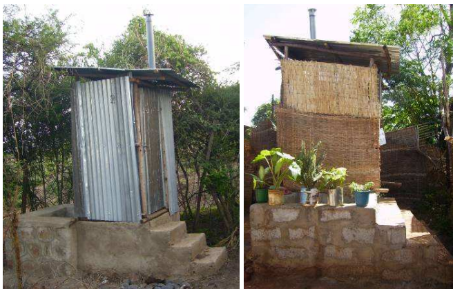
Fig. 7: Fossa alternas above ground (source: ROSA project Arba Minch, 2009)
