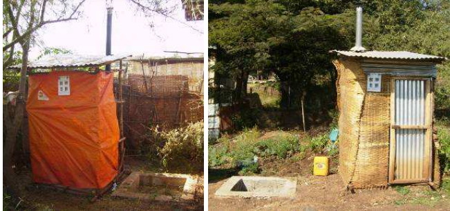
Fig. 6: Fossa alterna toilet superstructures (source: ROSA Project Arba Minch, 2008)
