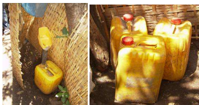
Fig. 9: Waterless urinal (source: ROSA project Arba Minch, 2009).
