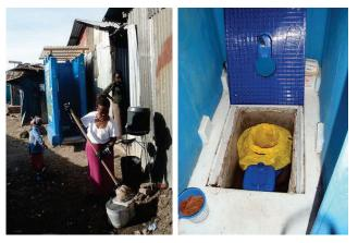
**Figure 53**. Left: 'Fresh Life' toilet, a UDDT with single vault for public use, with the franchise operator in a slum area of Nairobia, Kenya. Right: The interior of a 'Fresh Life' toilet with a removeable plastic slab with urine-diverting squatting pan (lifted up in the photo) and interchangeable containers for faeces and urine (photos: D. Mbalo, 2012).
