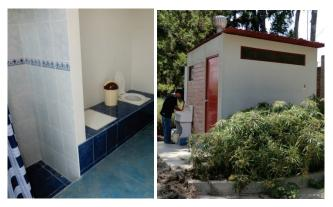
**Figure 35**. A bench UDDT with an attached shower for the security personnel at the university of Agraria de La Molina, Lima, Peru (photos: H. Hoffmann, 2011).
