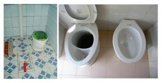
**Figure 7**. Left: Example in Kyrgyzstan with washing area in the centre of the photo, see arrow (photo: WECF, 2011). Right: Prototype of a ceramic urine-diverting pedestal in the Philippines with separate wash bowl for anal washing in a sitting position (photo: D. Lapid, 2007).
