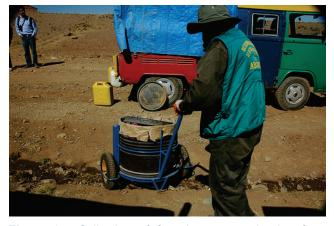
**Figure 37.** Collection of faecal matter and urine from UDDTs with single vaults in covered barrels and yellow containers, respectively, by the NGO Sumaj Huasi in El Alto, Bolivia (photo: A. Kanzler, 2009).
