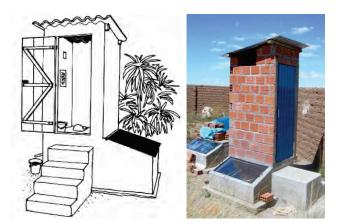
**Figure 25**. Left: Sketch of a UDDT with solar-heated processing vault (source: Winblad and Simpson-Hébert, 2004). Right: Solar heated UDDT installed in Bolivia (photo: R. Izurieta, 2011).
