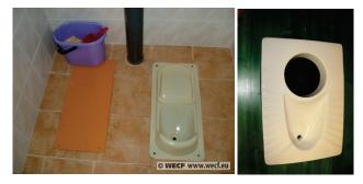
**Figure 8**. Left: Plastic urine-diverting squatting pan from China installed in a school in Ukraine (photo: WECF, 2010). Right: A ceramic urine-diverting squatting pan from *Tabor Ceramics* in Ethopia (photo: GIZ, 2009).
