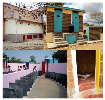
**Figure 56.** Top left: UDDTs in a school in Ukraine are attached to the school building, so that students can enter the restrooms from indoors (photo: WECF, 2006). Top right: A school near Machakos, Kenya with UDDT and attached boys urinal (photo: EPP, 2009). Bottom left: Girls urinals with UDDTs in Valalore secondary school in India. Bottom right: Detail of a squatting pan with anal washing section in a Sri Ramalingar secondary school in India (photos: NGO Wherever the Need, 2011).
