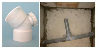
**Figure 27**. Left: Standard 45 degree coupling with inspection port (photo: internet source). Right: Two-inch plastic pipe inside a vault with sealed connections and slope exceeding 5%; the user interface with urine outlet pipe is placed from the top into the vertical pipe (photo: H. Hoffmann, 2010).
