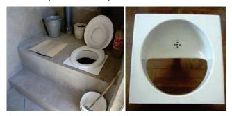
**Figure 6**. Left: Bench UDDT with single access step for sitting in Peru. Right: UD insert from *Rotaria del Peru<sup>11</sup>* in Peru (photos: H. Hoffmann, 2010).
