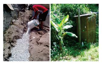
**Figure 43**. Left: Construction of a subsurface infiltration trench with gravel for greywater and urine at a school in Peru (photo: H. Hoffmann, 2009). Right: Urine is infiltrated next to an *Arborloo* in Zimbabwe (photo: P. Morgan, 2007).
