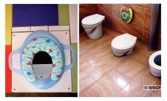
**Figure 34**. Left: A movable child seat adapter for a bench design in Peru (photo: H. Hoffmann, 2009). Right: Lowered UD pedestals for children at a school in Georgia (photo: WECF, 2010).
