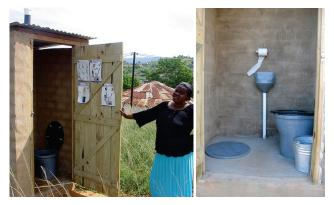
**Figure 52**. Left: Exterior view of a double vault UDDT in a peri-urban area of the eThekwini Municipality, South Africa (photo: eThekwini Water & Sanitation Unit, 2005). Right: Interior view of a similar toilet in eThekwini Municipality (photo: E. v. Münch, 2005).
