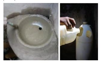
**Figure 33.** Left: Example of a simple concrete hand washing basin inside a toilet cubicle. Right: A simple water dispenser made from a 5-litre plastic bottle (photos: A. Shangwa, 2010).
