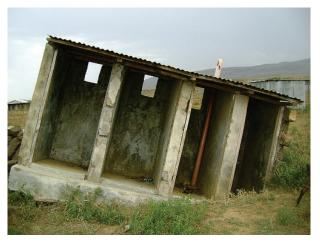
**Figure 3**. A collapsed pit latrine in Narok, Kenya, built on unstable sandy soil that could not withstand the rain events (photo: P. Mboya, 2009).
