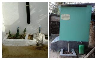
**Figure 31**. Left: A planted soak pit for anal wash water with a container for urine collection in India (photo: L. Dengel, 2009). Right: An unplanted soak pit filled with crushed brick in Bangladesh (photo: M. Alam, 2011).
