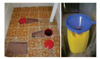
**Figure 51**. UDDT interface made from pipe and moulded urine section by WECF (photo: S. Deegener, 2010). A waterless urinal from the ROSA project in Arba Minch, Ethopia (photo: R. Ingle, 2009).
