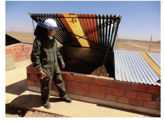
**Figure 40**. The Bolivian NGO Sumaj Huasi is vermicomposting faeces with subsequent solar drying in the same compartment in El Alto, Bolivia (photo: H. Hoffmann, 2012).
