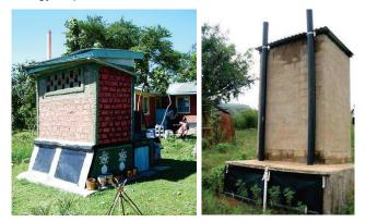
**Figure 24.** Left: UDDT with slightly inclined metal vault doors in Kenya (photo: C. Rieck, 2010). Right: Toilet in eThekwini Municipality, South Africa with vertical sliding plastic doors (photo: eThekwini Water & Sanitation Unit, 2009).
