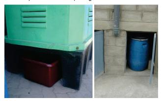
**Figure 22.** Left: Pre-fabricated plastic UDDT, called an EKO-LOO<sup>16</sup> with one interchangeable faeces container from *Kentainers* in Kenya (photo: C. Rieck, 2008). Right: Use of a plastic drum in a toilet for students at Adama University in Ethopia. The tight fitting lid is used for transport of the full drum (photo: K. M. Sintayehu, 2010).
