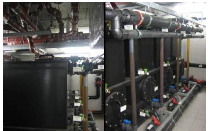
Fig. 5: Left: Plastic urine storage tanks in the basement of House 1 with connected urine pipework. Right: urine tanks with level indicating plastic pipes (source: L. Ulrich, April 2009).
