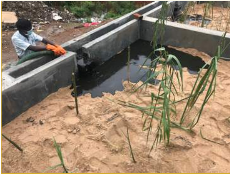
FIGURE 6 FEEDING OF FAECAL SLUDGE INTO VERTICAL WETLAND
