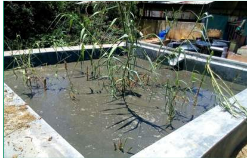
FIGURE 7 VERTICAL WETLAND AFTER FEEDING OF FAECAL SLUDGE
