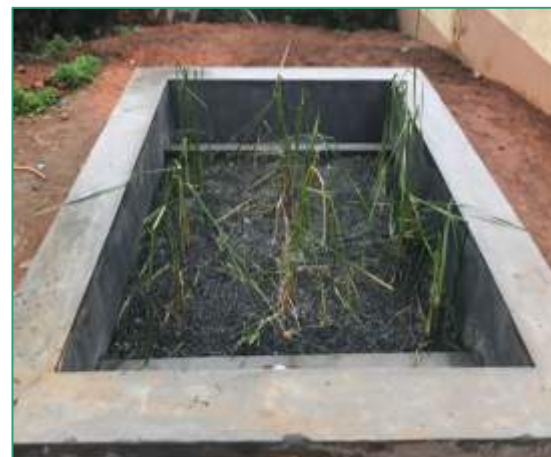
FIGURE 9 HORIZONTAL CONSTRUCTED WETLAND (VIEW FROM THE TOP)
