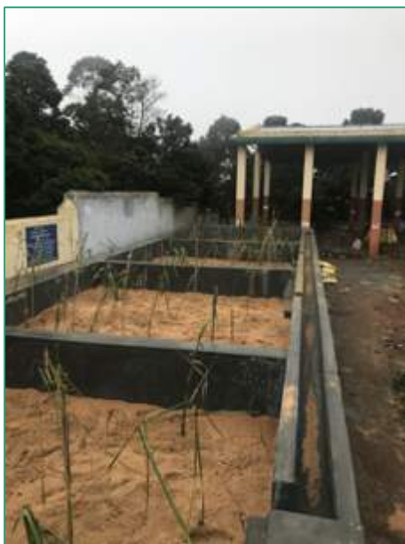
FIGURE 4 VERTICAL CONSTRUCTED WETLAND
