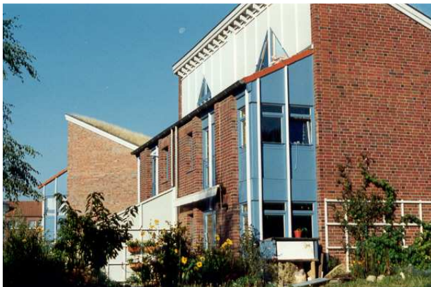
Fig. 5: Houses with green roof in northern courtyard, constructed in 1990/91 (source: Berger Biotechnik).
