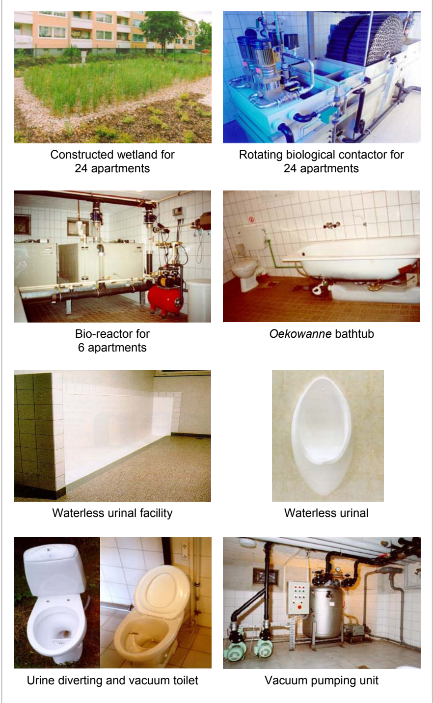
Figure 2: Innovative Technologies installed in the Oeko-Technik-Park (photo: Oeko-Technik-Park)
