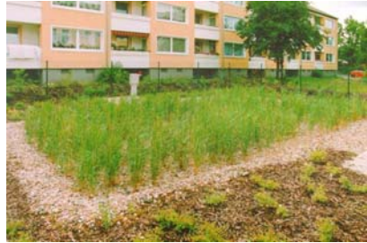
Constructed wetland for 24 apartments
