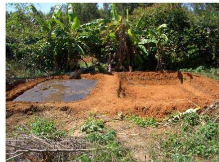
fig. 6: Sludge drying beds. (source: seecon gmbh)
