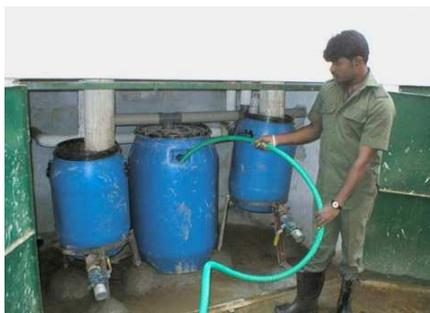
fig. 3 and 4: Evacuation of faecal matter with the newly installed vacuum system (top). Emptying of urine collection tanks (bottom). (source: seecon gmbh)
