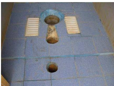
fig. 2: Squatting slab provided with 3 holes. (source: seecon gmbh)
