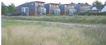
Figure 1: Twin houses in Flintenbreite (source: GTZ)
