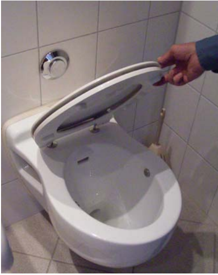
Figure 3: Vacuum toilet (source: Otterwasser)
