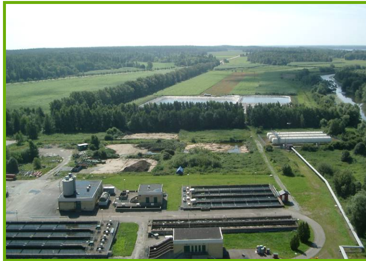
Picture 25. SRP wastewater system Enköping / Sweden. [Photo by: I. Dimitriou, SLU]
