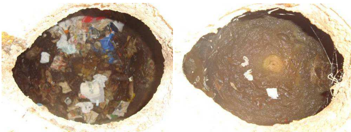
Figure 3.3 Two pits from the Mafunze study, showing high and low rubbish levels
