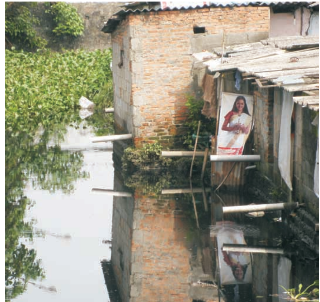
Figure 34: Clogging of storm drains
