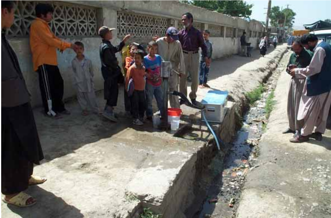
Fig. 3.62: A hand-pumped well extracting shallow groundwater in an urban district of Kabul immediately adjacent to an open sewage channel (photo: TÜNNERMEIER).
