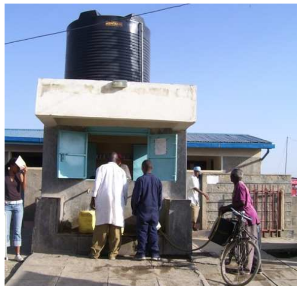
Fig. 5: Customers of the water kiosk. The water tank on the roof holds 5 m 3 (or 250 jerry cans) to bridge water supply gaps for a period of about 1-2 days.
