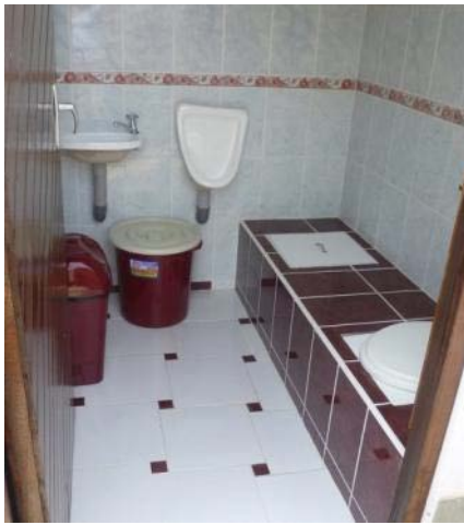
Figure 2: Double vault bench UDDT in Lima, Peru with a waterless urinal and wide bench UDDT on the right. It could be easily adapted for users with disabilities e.g. by adding handrails and allowing more space (source: H. Hoffmann, 2010).
