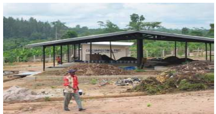
Fig. 3: Co-composting facility (open windrow system) in Kumasi (source: IWMI, 2003).
