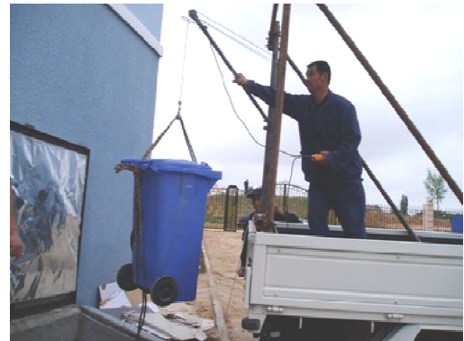
Fig. 8: Removal of basement faeces bins by using a simple hoist installed on a light truck (source: SEI).
