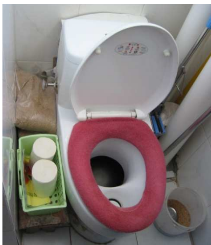
Fig. 10: Private bathroom with urine diversion dry toilet pedestal (source: C. Olt, 2008).
