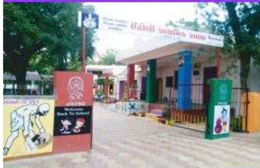
LANTOLI PRIMARY SCHOOL, VADODARA GUJARAT
