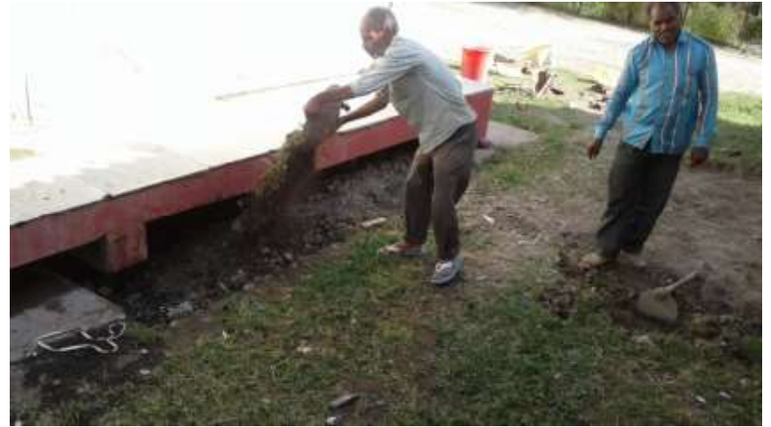
Cleaning and covering the gaps
