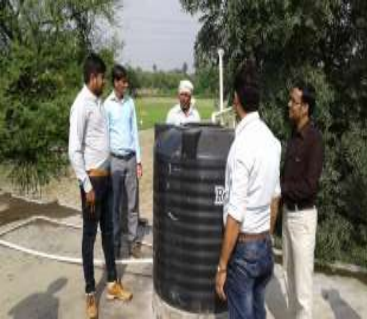
Over Head Tanks (Before intervention)
