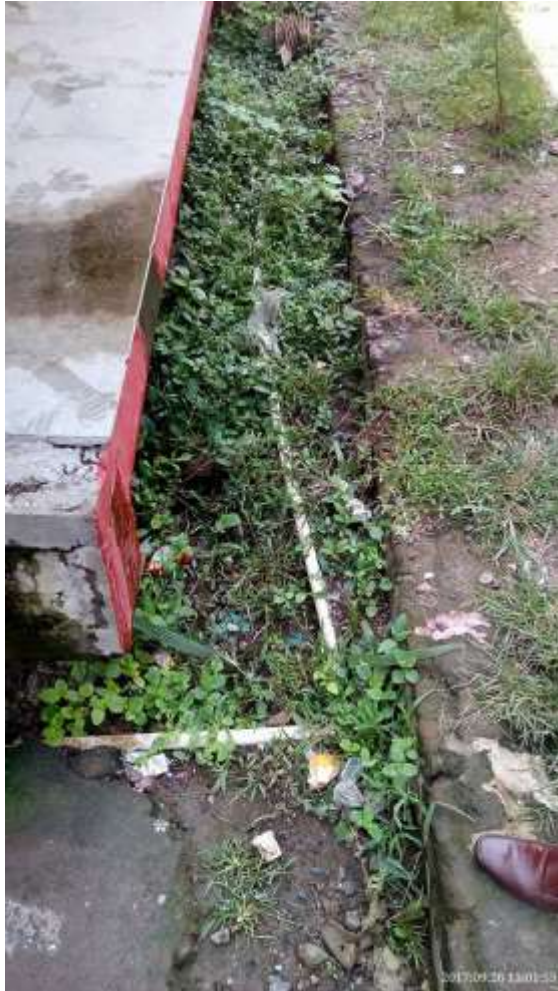
Water pipe line passing through a flooded area
