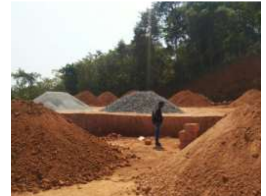
Material Recovery Facility under final phase of construction in Ramanagara and Dakshina Kannada
