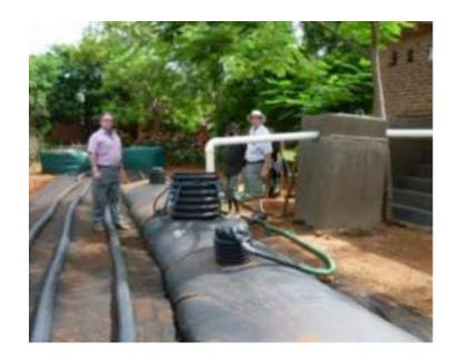
'Flexigester' Anaerobic Digester
