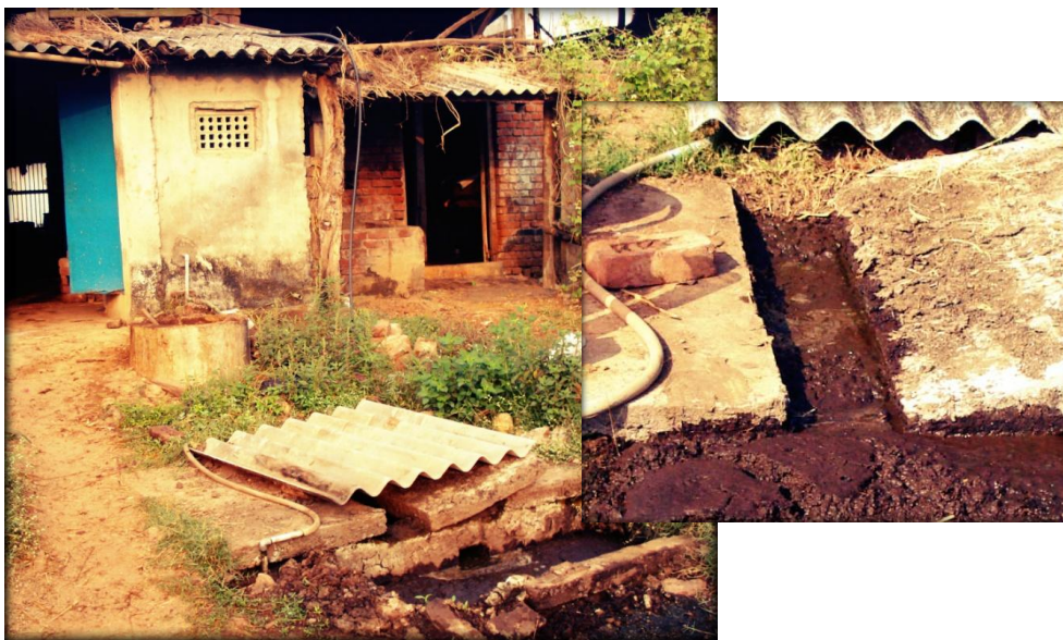
Figure 3-6 Slurry at the outlet of toilet linked biogas plant
