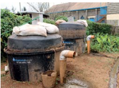
Biodigester Source: Takamoto Biogas
