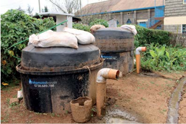
Biodigesters. Source: Takamoto Biogas
