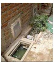
Figure 2: Until 2007 UDDT in Lima always mixed grey water with urine, but the infiltration often didn't work properly. Source: P.Oswald
