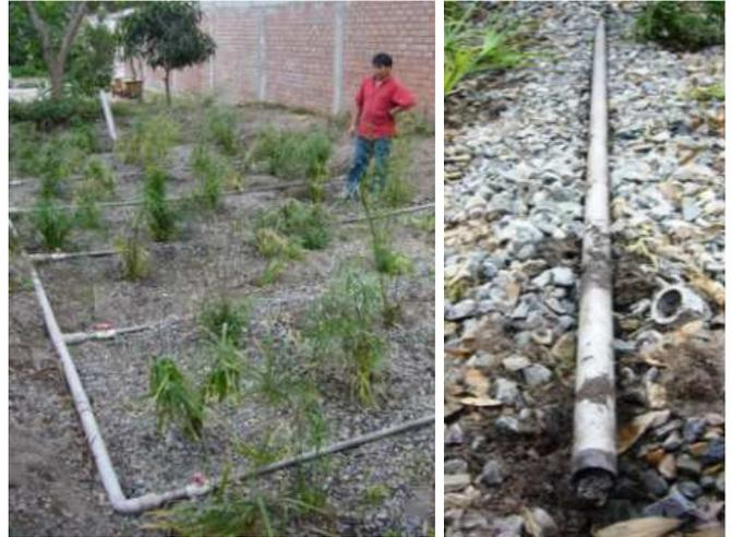
Figure 29. Left: cleaning the wastewater distribution pipes by opening and closing valves and caps during the pumping phase (medium sized papyrus umbrella sedge plants just after re-planting). Right: opened cap on a blocked distribution pipe (photos of VFB for blackwater treatment at school in Lima, Peru by H. Hoffmann, 2009)
