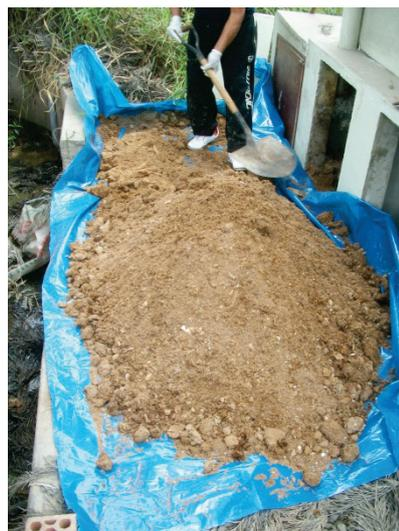
**Figure 18.** Emptying of dehydrated faecal material from a double vault UDDT after 6 months of storage at the university of Agraria de La Molina, Lima, Peru (photo: H. Hoffmann, 2011).
