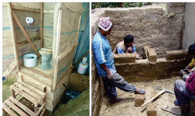
**Figure 50.** Left: Low-cost model of a UDDT with single vault system in the Philippines (photo: R. Gensch, 2009); Right: Low-cost UDDT built with adobe bricks in Peru (photo: H. Hoffmann, 2009).
