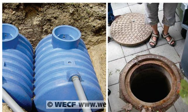
**Figure 29.** Left: Underground plastic urine storage tanks in Ukraine (photo: WECF, 2009). Right: Concrete urine storage tank in Sweden (photo: E. v. Münch, 2007).
