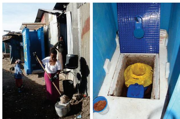
**Figure 53.** Left: 'Fresh Life' toilet, a UDDT with single vault for public use, with the franchise operator in a slum area of Nairobi, Kenya. Right: The interior of a 'Fresh Life' toilet with a removable plastic slab with urine-diverting squatting pan (lifted up in the photo) and interchangeable containers for faeces and urine (photos: D. Mbalo, 2012).
