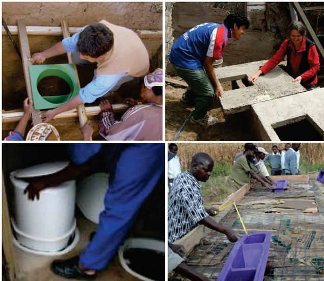
**Figure 14.** Top left: Placing a urine-diverting insert for a bench slab made of adobe in Peru (photo: H. Hoffmann, 2009). Top right: Precast concrete bench slab in Peru (photo: H. Hoffmann, 2011). Bottom left: Pedestals fixed with a socket system, manufactured by *Envirosan Ltd.* in South Africa (photo: B. Lewis, 2008). Bottom right: Placement of plastic twin drop-hole squatting pan prior to casting reinforced concrete slab in Kenya (photo: W. Osumba, 2010).
