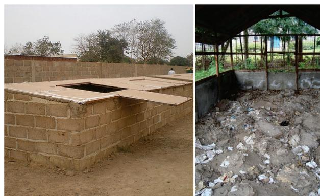
**Figure 41.** Left: Prolonged storage of dry faeces from double dehydration vaults in Burkina Faso (photo: A. Fall, 2009). Right: Drying shed with faecal matter from single vaults in Kenya (photo: L. Kraft, 2011).
