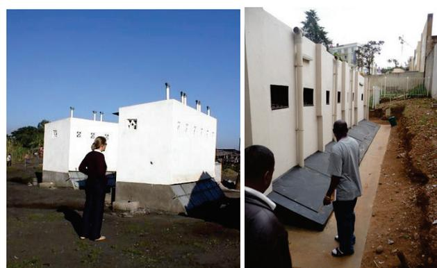
**Figure 59.** Left: A public toilet with integrated showers built by *the Austrian Red Cross* at a market place in Mozambique (photo: M. Fogde, 2006). Right: Rear view of underground single vaults of public toilet at UTC roundabout in Kigali, Rwanda (photo: L. Dagerskog, 2011).
