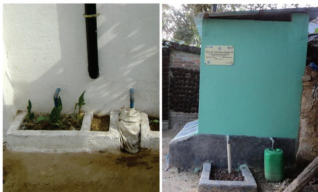
**Figure 31.** Left: A planted soak pit for anal wash water with a container for urine collection in India (photo: L. Dengel, 2009). Right: An unplanted soak pit filled with crushed brick in Bangladesh (photo: M. Alam, 2011).
