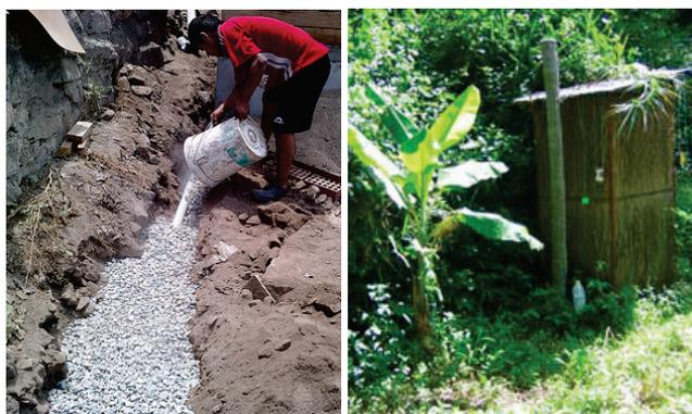
**Figure 43.** Left: Construction of a subsurface infiltration trench with gravel for greywater and urine at a school in Peru (photo: H. Hoffmann, 2009). Right: Urine is infiltrated next to an *Arborloo* in Zimbabwe (photo: P. Morgan, 2007).
