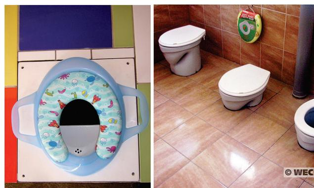
**Figure 34.** Left: A movable child seat adapter for a bench design in Peru (photo: H. Hoffmann, 2009). Right: Lowered UD pedestals for children at a school in Georgia (photo: WECEF, 2010).
