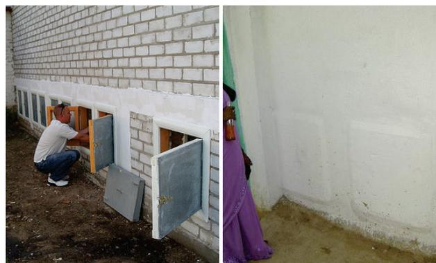
**Figure 23.** Left: Wood frame doors with metal cover sheeting at a school in Ukraine (photo: WECF, 2010). Right: Semi-permanent brick and mortar doors for a household UDDT with double dehydration vaults in India (photo: L. Dengel, 2009).
