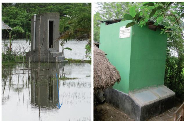
**Figure 60.** Left: A UDDT with vault doors elevated above the flood line (photo: A. Delepière, 2009). Right: Detail of raised access vault doors that prevent water entry into the dehydration vaults (photo: M. Alam, 2011).
