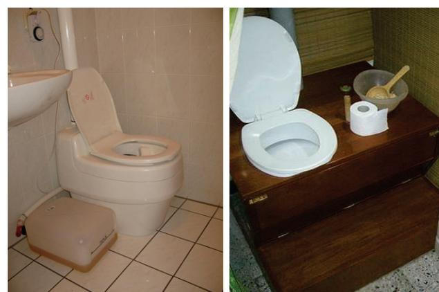
**Figure 55.** Left: Indoor urine diversion dry toilet with single vault and electrical ventilation manufactured by *Separett* (photo: E. v. Münch, 2008). Right: A single vault UDDT with wooden bench and interior vault door built by *Rotaria del Peru* in Lima, Peru (photo: H. Hoffmann, 2010).
