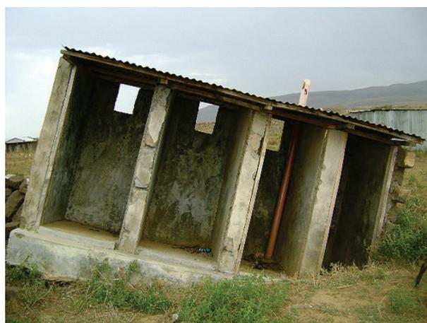
**Figure 3.** A collapsed pit latrine in Narok, Kenya, built on unstable sandy soil that could not withstand the rain events (photo: P. Mboya, 2009).
