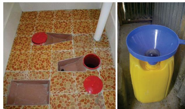
**Figure 51.** UDDT interface made from pipe and moulded urine section by WECF (photo: S. Deegener, 2010). A waterless urinal from the ROSA project in Arba Minch, Ethiopia (photo: R. Ingle, 2009).
