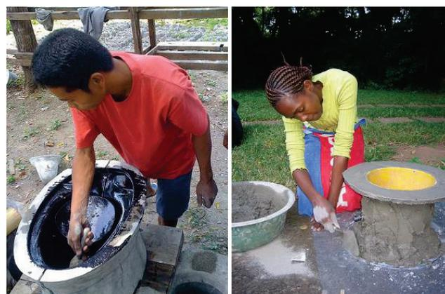
**Figure 12.** Left: Casting of concrete pedestals using professional moulds in the Philippines (photo: R. Gensch, 2010). Right: Moulding a concrete pedestal around a bucket, with a plastic urine separation fitting (photo: P. Morgan, 2008).
