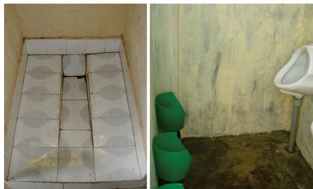
**Figure 11.** Left: Tiled, waterless squatting urinal installed in a female toilet at a secondary school in Nakuru, Kenya. (photo: M. Wafler, 2010). Right: Wall-mounted male urinals made from plastic buckets and from standard ceramic bowls for different age groups in a church and pre-school in Nakuru, Kenya (photo: E. Müllegger, 2009).
