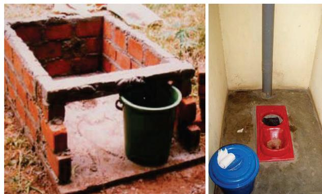
**Figure 21.** Left: Single vault under construction in Zimbabwe that can easily fit two or more containers (photo: P. Morgan, 2007). Right: Interior of a UDDT with a single vault in Kampala, Uganda (photo: E. Schröder, 2010).
