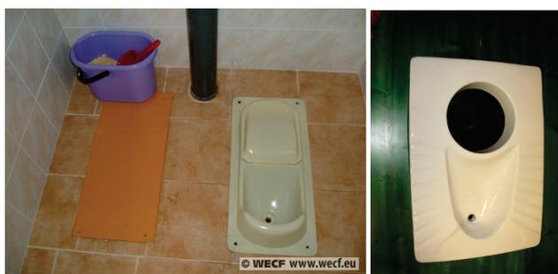
**Figure 8.** Left: Plastic urine-diverting squatting pan from China installed in a school in Ukraine (photo: WECF, 2010). Right: A ceramic urine-diverting squatting pan from Tabor Ceramics in Ethiopia (photo: GIZ, 2009).
