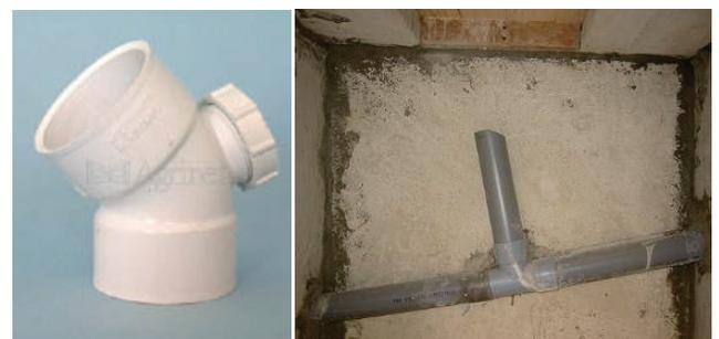
**Figure 27.** Left: Standard 45 degree coupling with inspection port (photo: internet source). Right: Two-inch plastic pipe inside a vault with sealed connections and slope exceeding 5%; the user interface with urine outlet pipe is placed from the top into the vertical pipe (photo: H. Hoffmann, 2010).
