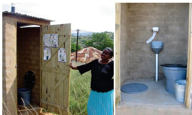
**Figure 52.** Left: Exterior view of a double vault UDDT in a peri-urban area of the eThekweni Municipality, South Africa (photo: eThekweni Water & Sanitation Unit, 2005). Right: Interior view of a similar toilet in eThekweni Municipality (photo: E. v. Münch, 2005).
