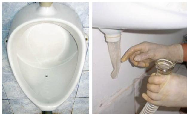
**Figure 15.** Left: Flushing ceramic urinal retrofitted for waterless use by sealing all but a single drainage hole. Right: Condom with cut-off tip attached to the urinal outlet as an odour control measure at the user interface level (photos: C. Wendland, 2010).
