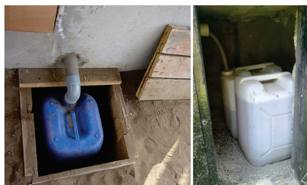
**Figure 28.** Left: Urine discharge into 20L plastic container (photo: H. Hoffmann, 2009). Right: 20L collection container in an additional vault in Zambia; note the insufficient hose diameter (photo: R. Ingle, 2010).
