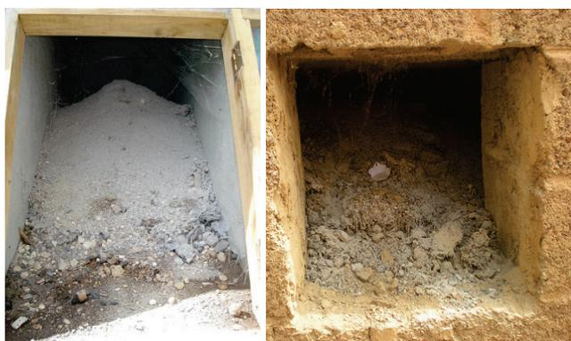
**Figure 17.** Left: Dried faeces with ash cover inside the vault of a UDDT in the Philippines (photo: E. Sayre, 2008). Right: Dehydration vault with soil and ash cover in Burkina Faso (photo: S. Tapsoba, 2009).
