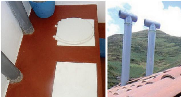
**Figure 26.** Ventilation piping in Peru with inside installation and a vent cover with T-joints (source: H. Hoffmann, 2010).
