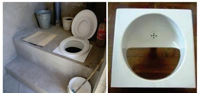
**Figure 6.** Left: Bench UDDT with single access step for sitting in Peru. Right: UD insert from *Rotaria del Peru*<sup>11</sup> in Peru (photos: H. Hoffmann, 2010).
