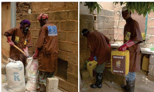
**Figure 48.** Left: Emptying the inactive vault of a UDDT after a six-month storage period in Ouagadougou in Burkina Faso. Right: Emptying the urine containers in Ouagadougou (photos: S. Tapsoba, 2009).
