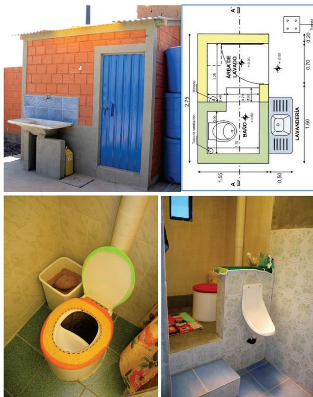
**Figure 54.** Top: A bathroom building with shower, urinal and a UDDT with single vault in El Alto, Bolivia (photo: S. Frenzel, 2012 and source: Suntura et al., 2012). Bottom: Interior of the toilet with UD pedestal (left), urinal and shower in the foreground and two access steps leading to toilet in the background (photos:K. Andersson, 2011).
