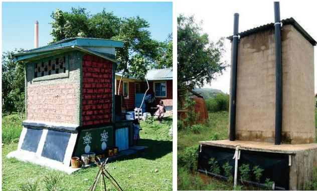
**Figure 24.** Left: UDDT with slightly inclined metal vault doors in Kenya (photo: C. Rieck, 2010). Right: Toilet in eThekweni Municipality, South Africa with vertical sliding plastic doors (photo: eThekweni Water & Sanitation Unit, 2009).
