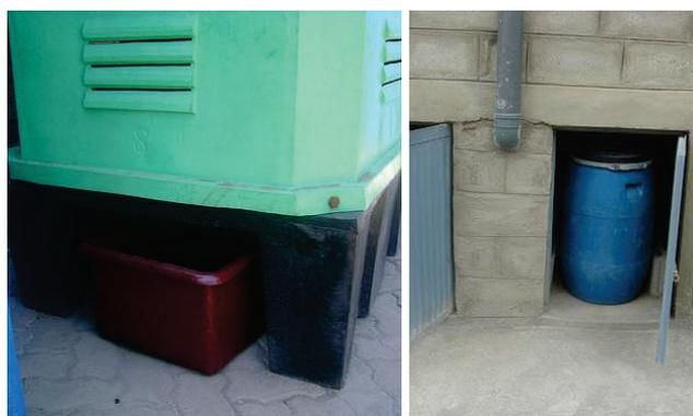
**Figure 22.** Left: Pre-fabricated plastic UDDT, called an EKO-LOO<sup>16</sup> with one interchangeable faeces container from *Kentainers* in Kenya (photo: C. Rieck, 2008). Right: Use of a plastic drum in a toilet for students at Adama University in Ethiopia. The tight fitting lid is used for transport of the full drum (photo: K. M. Sintayehu, 2010).
