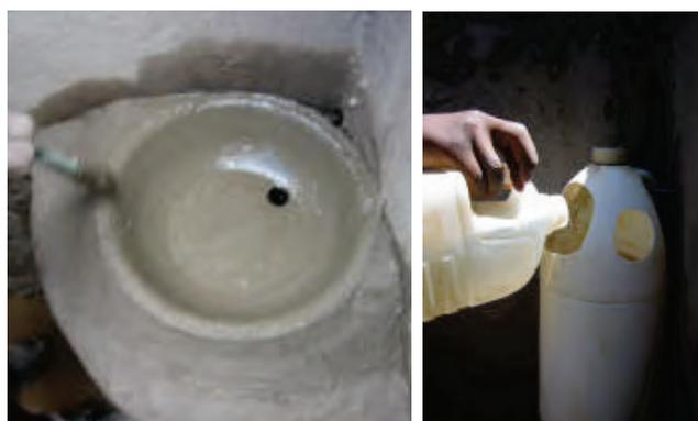
**Figure 33.** Left: Example of a simple concrete hand washing basin inside a toilet cubicle. Right: A simple water dispenser made from a 5-litre plastic bottle (photos: A. Shangwa, 2010).
