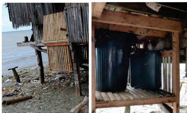
**Figure 61.** A hanging single vault urine-diverting dry toilet at a shore line area in the Philippines<sup>44</sup> (photos: R. Gensch, 2010).
