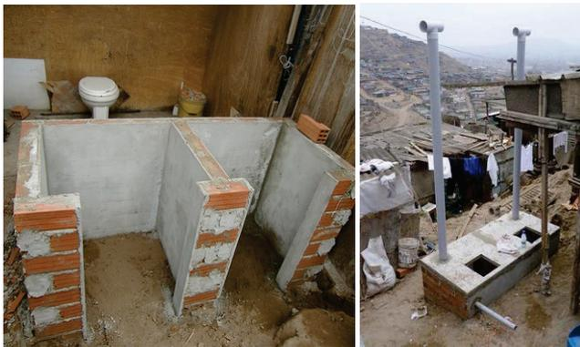
**Figure 19.** Left: Dehydration vaults under construction in Peru (photo: H. Hoffmann, 2011). Right: A dehydration vault on sloping terrain is built partially below the ground (photo: H. Hoffmann, 2011). Both toilets are still under construction here.
