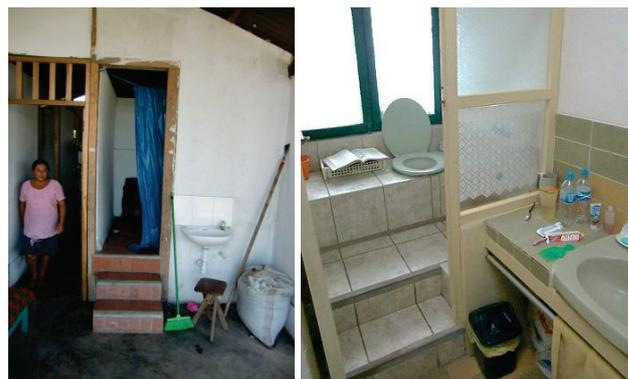
**Figure 32.** Examples of indoor UDDTs with bench design being integrated houses and even existing bathrooms (photos: H. Hoffman, 2011).
