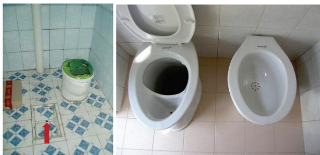
**Figure 7.** Left: Example in Kyrgyzstan with washing area in the centre of the photo, see arrow (photo: WECF, 2011). Right: Prototype of a ceramic urine-diverting pedestal in the Philippines with separate wash bowl for anal washing in a sitting position (photo: D. Lapid, 2007).
