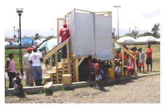
Figure 1: Raised toilets in Haiti provided by IFRC for 275,000 people per day with materials produced in Dominican Republic and constructed in Haiti (source: IFRC, 2010).
