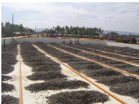
Fig. 5: Preparation of drainage system of cell 1 of the constructed wetland (vertical flow), January 2006 (source: DILG-GTZ Program).
