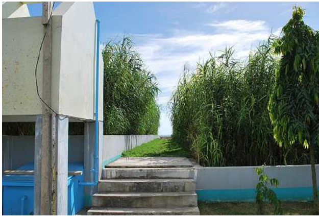
Fig. 10: Constructed wetland in Bayawan city. The space is between the vertical and the horizontal flow subsurface flow bed (source: J. Boorsma, 2009).
