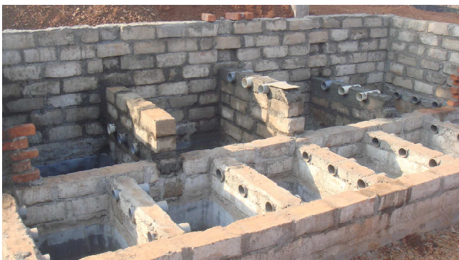
Fig. 6: Construction of ABR and UF (photo: N. Zimmermann)
