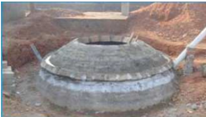
Fig. 5: Biogas settler (under construction) (photo: N. Zimmermann)
