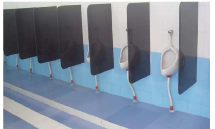
Fig. 8: Waterless urinals for boys (photo: N. Zimmermann)
