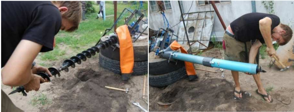
Figure 4.8 Adding an extension to the auger
