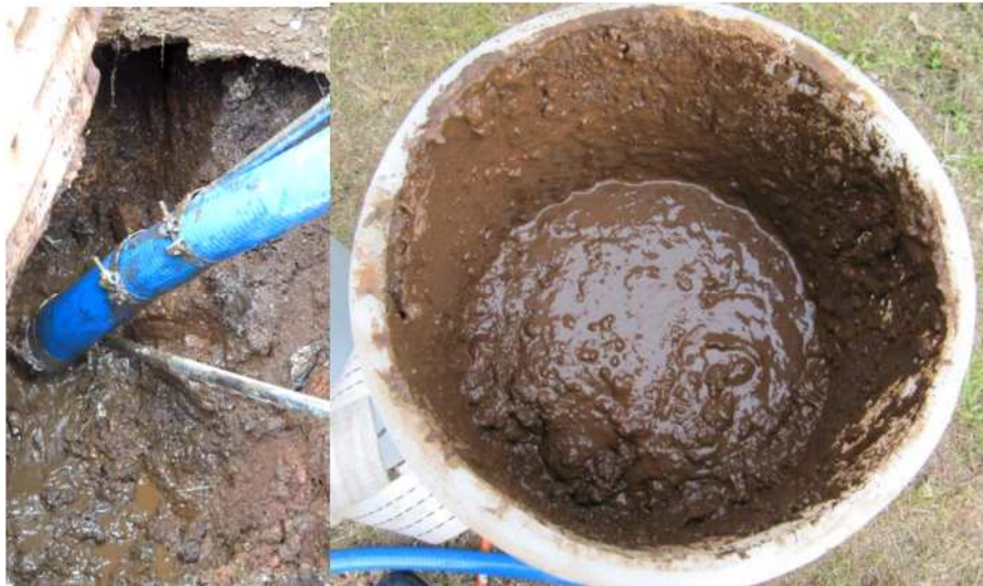
Figure 7.11 Emptying a pit with the eVac
