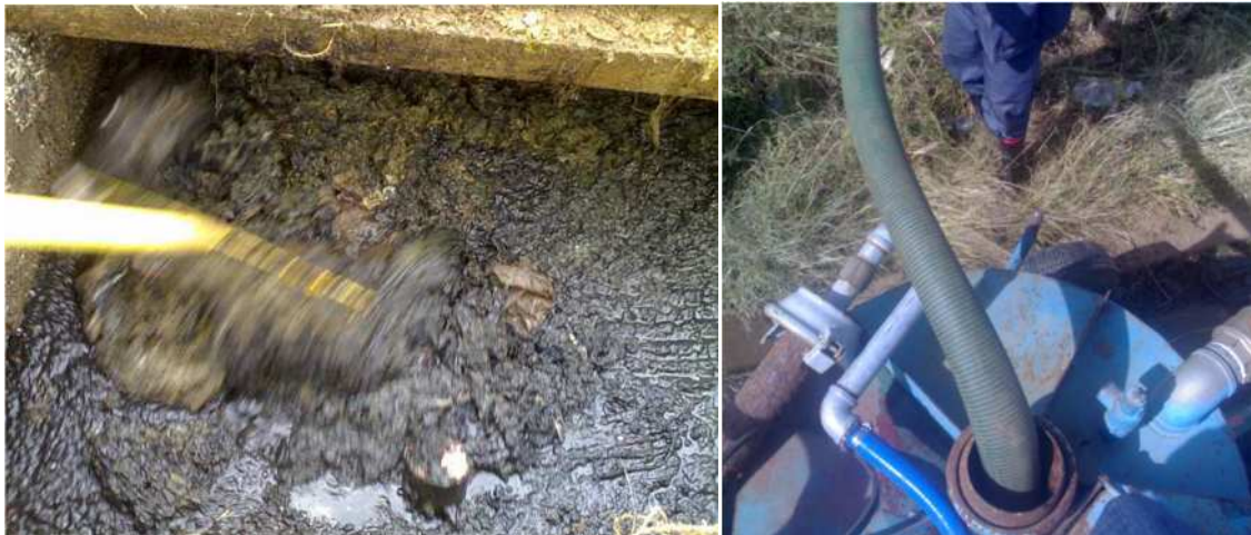
Figure 5.11 Rubbish being removed from a pit with a rake (left). Using the Vacutug hose to mix water with sludge inside the tank (right).
