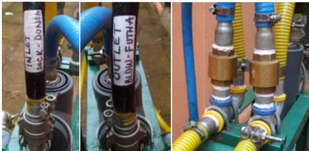
Figure 6.5 Colour coding and labelling to aid correct operation
