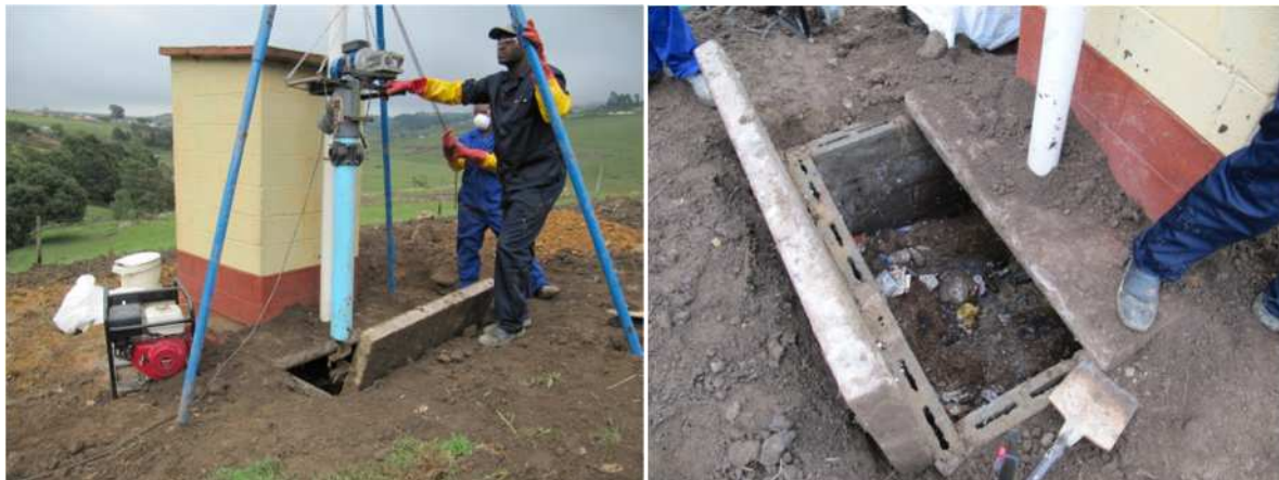
Figure 4.11 Using the auger to empty a VIP pit (left). The amount of rubbish which the pit contained (right) made it impossible for the auger to remove sludge.
