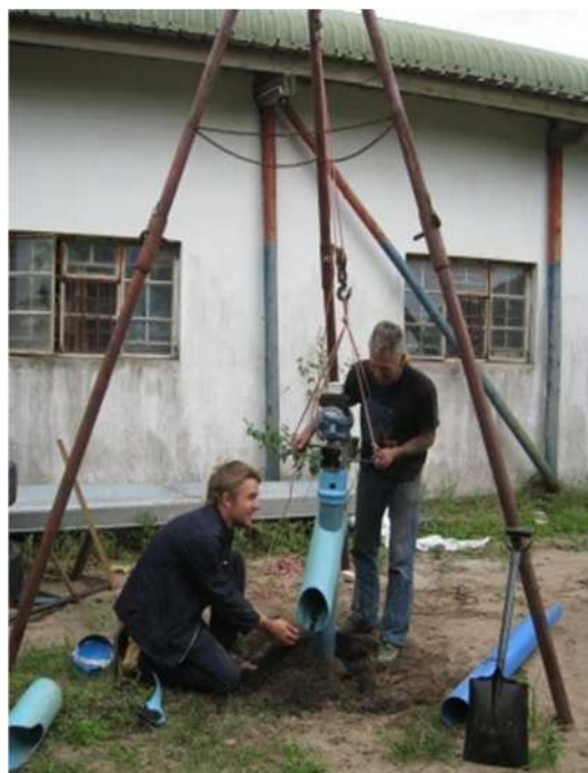
Figure 4.9. Using a tripod to support the Pit Sludge Auger while it is manoeuvred around the sludge
