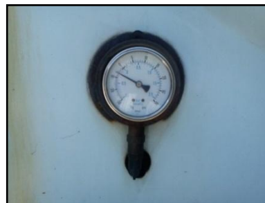
(f): Pressure scale that shows real time pressure during operation of FS emptying system. Usually, there is no adjustment of pressure during operation except for when there is difficulty that requires high pressure of vacuum system.
