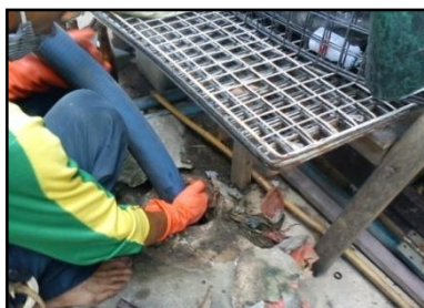
(k): Another person is responsible for controlling level of hose-ended and makes sure that all of FS is sucked out from septic tank.
