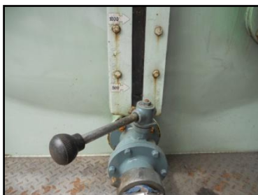
(m): Sludge level in the tank is shown on scale.
