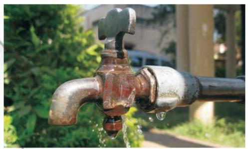
Figure 22: Leaking public standpost
