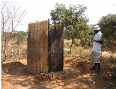
**A series of hardwood or treated poles has been placed around the slab in holes drilled by an earth auger. Three wires have been tightly wrapped around the holes for attachment of the cleaned grass. The grass is attached to the poles as bundles. A disc of strong concrete can be made to fit over the ventilation pipe hole before a pipe is fitted. A vent pipe can be fitted later**
