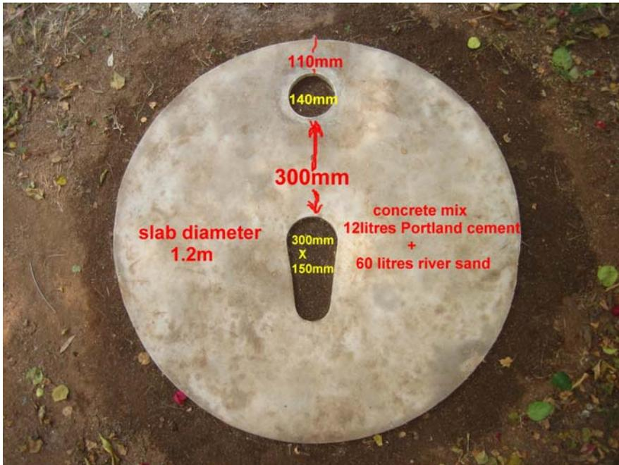
Details of concrete slab for uBVIP
