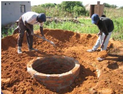
The pit lining extends about 20cm above ground level. The annular space between the dug pit and the pit lining being filled in.
