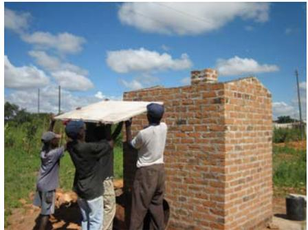
The four panels are allowed to cure for at least 7 days being kept wet at all times. Each panel is carefully lifted from the plastic sheet and placed on the superstructure in the appropriate place, embedded in cement mortar.
