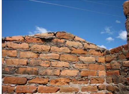
The walls are built up. The end walls and mid wall which will support the roof are built up so the roof will slope outwards.
