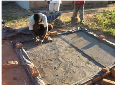
**A sheet of plastic is best laid on the ground to cover the soil within the brick mould. The cement will loose less moisture when laid over plastic and will develop more strength. The mix of cement is laid in sections. The mix of cement is 4 parts river sand to 1 part PC15 cement. To make the roof 3 mixes of 12li cement and 48li river sand (4:1) were used.**
