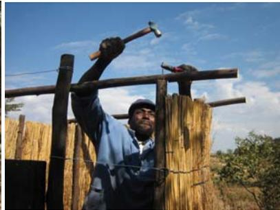
**The roof is prepared for attachment to the grass and pole structure. Extra poles are added to the upright poles for attachment to the roof.**
