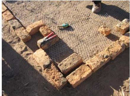
**An area of ground is levelled and a mould made with bricks to suit the size of the roof required. In this case the total area was 2m X 1.8m. The chicken is laid within the mould and cut up into four pieces (900mm x 870mm (2 pieces) and 900mm x 1130mm (2 pieces)). The exact measurements should be taken from the structure, which varies slightly in each case. A recess was made in one of the four panels for the vent pipe.**
