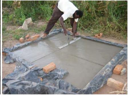
Each section is covered with a layer of cement about 20mm thick and the wire is laid over this to cover the section. The wire is then covered with another layer of cement. Later on the concrete will be cut with a trowel when still soft. The sections of wire in the concrete must be separated clearly so the trowel cuts through concrete only. The concrete is then covered for the night. It is watered the following morning and kept wet and covered for a week before moving on to the structure.
