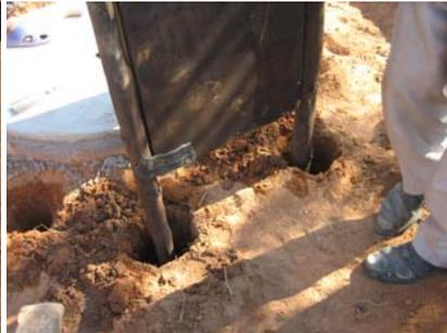
**Fitting a car rubber hinge to one of the treated gum poles. The final pole and door unit ready to mount in front of the slab. The two holes drilled for the two main “king posts” are drilled in front of the slab. The door should be about 65cm in front of the squat hole and door posts 50cm apart.**
