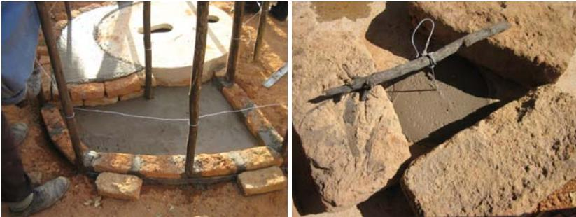
**Extension of the concrete floor made at the entrance. The vent hole can be plugged or capped with a concrete plug.**
