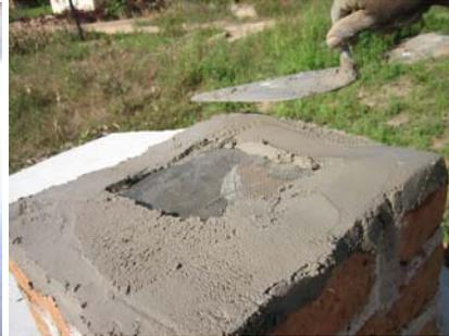
**All the internal surfaces of the Blair VIP are plastered. The floor is also dished to allow drainage of water into the brick lined pit. A fly screen made of aluminium is then embedded in cement mortar to the top of the vent pipe**
