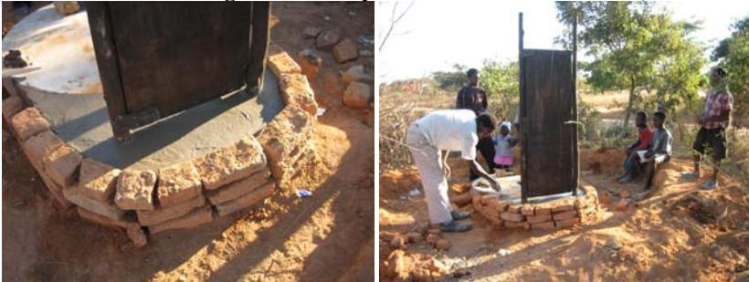
**This door unit can be linked to a grass and pole structure or linked to brickwork. The following photos show the link to poles and grass.**
