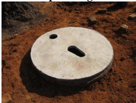
Weak mortar is laid around the rim of the pit lining. The slab is then mounted. The orientation of the slab depends on the type of structure to be built. In this case a square spiral structure will be built, so the pipe hole will be on the same side as the toilet structure opening.
