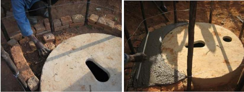
**Poles are placed around the slab in a spiral shape. Cement left over from the pit lining is used to make a cement floor in front of the slab. This cement can be extended into the entrance of the toilet**
