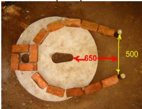
The distances between poles (500mm) and between the door and the squat hole (650mm)
