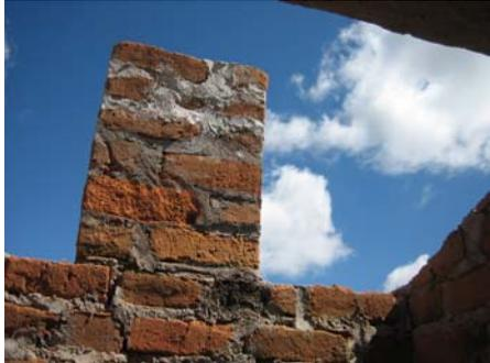
The vent pipe is raised 6 courses above the wall level. Later it is fitted with a corrosion resistant fly screen.
