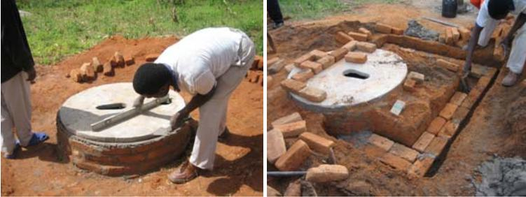
The slab is made level on the elevated brickwork above ground level and the weak cement mortar smoothed down around the slab so the slab and brick lining are airtight. The slab and pit must have an airtight fit of the vent pipe to work properly. A trench is cut down in the soil around the toilet. The brick foundation for the walls will be laid in this following the dimensions below,
