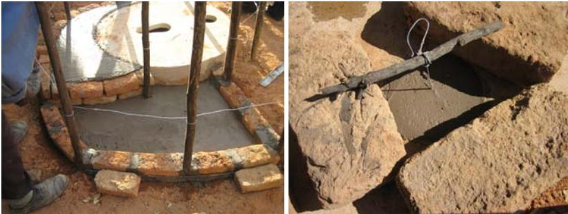
**Extension of the concrete floor made at the entrance. The vent hole can be plugged or capped with a concrete plug.**
