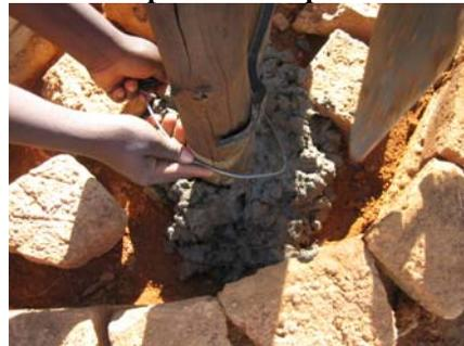
**A mould made of bricks is built up around the two main poles. This is filled with a mix of broken bricks, stones and concrete to anchor the posts. Each post is surrounded by a ring of steel wire.**
