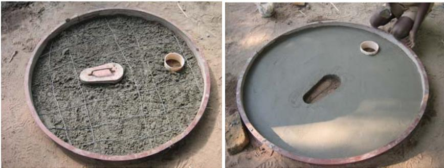
Making the concrete slab for the uBVIP. Half the concrete mix is added first. Then the wire reinforcing is added. Then the remainder of the concrete is added and smoothed down flat.
