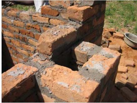
Walls and vent come up together. The walls are built up to 1.8m in height and the pipe to about 2.4m, The internal surfaces of the brickwork inside the pipe must be kept smooth.
