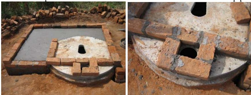
**The walls are built up together with the vent pipe as shown**
