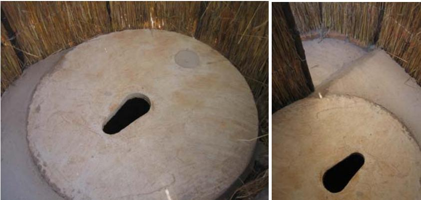
**The concrete floor is extended in front of the slab and also within the entrance.**
