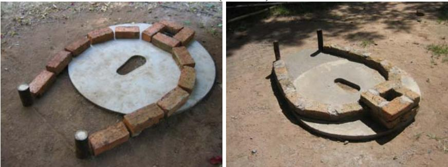
One arrangement for the brick structure is to construct it in a horseshoe shape and connected the bricks to the two poles (king posts). The toilet floor is extended in front of the round slab around the poles. The horseshoe shaped structure is very easy to build and has been called the “horseshoe Blair.” It derives strength from its shape. It can also be fitted with a tubular pipe.
