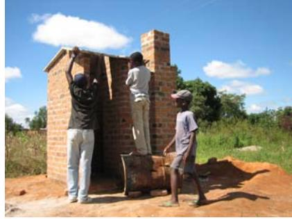
**Each panel is supported by the dividing wall in the centre of the structure as shown**
