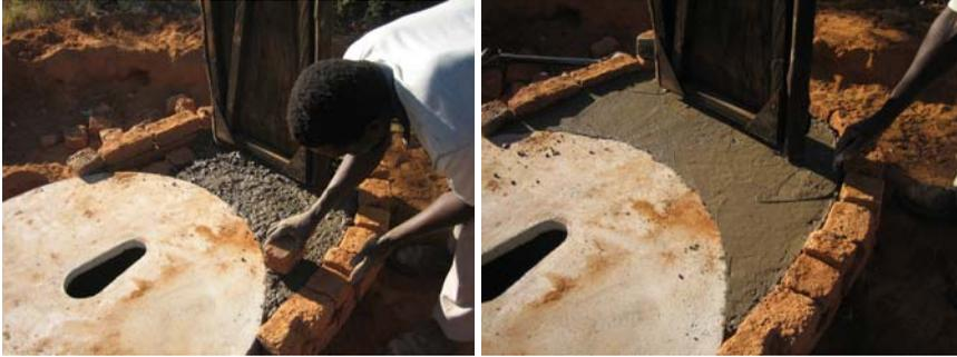
**The concrete mix is built up inside the brick mould to slab level. This is left to cure overnight before any further work commences,**
