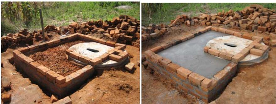
The brick walls are laid on the foundation so the outer dimensions of the brick walls are close to 1.45m X 1.85m. The walls are built up to slab level. The toilet floor area is then backfilled with brick rubble to lower slab level. This is then filled with a concrete mix (10 litres cement + 50 litres river sand).
